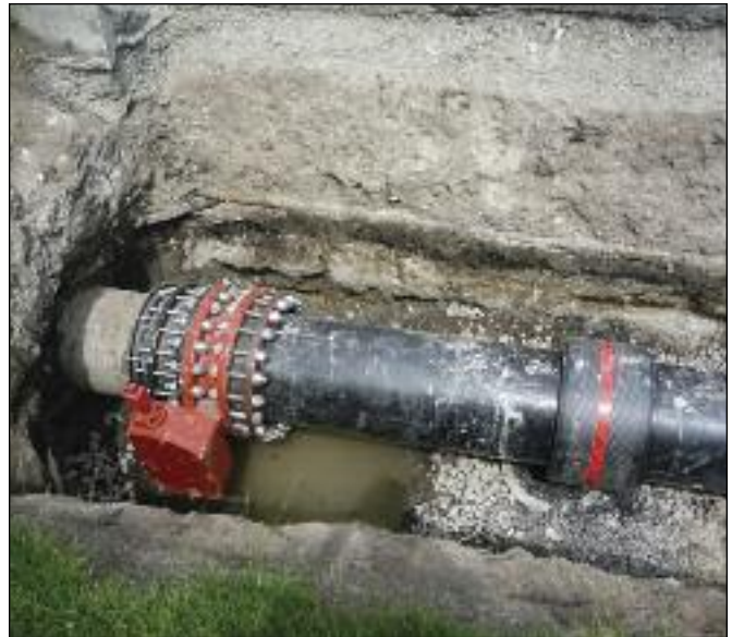
Final tie-in at pit using a liner grip fitting, butterfly valve, and electrofusion coupler
