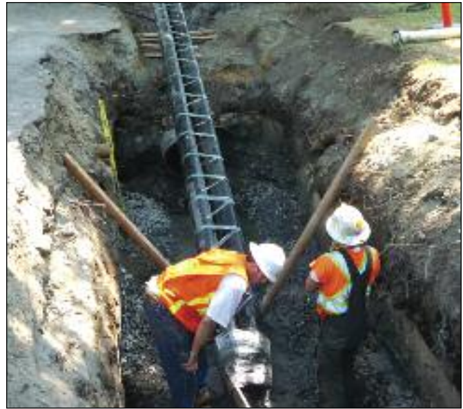
Liner insertion at entry pit
