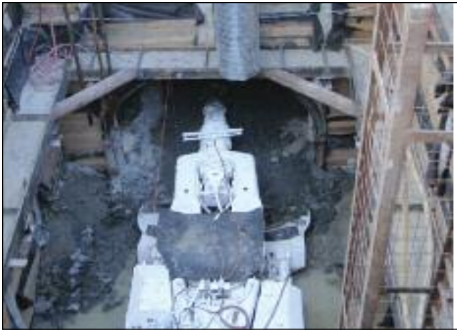
The start of Tunnel Excavation
