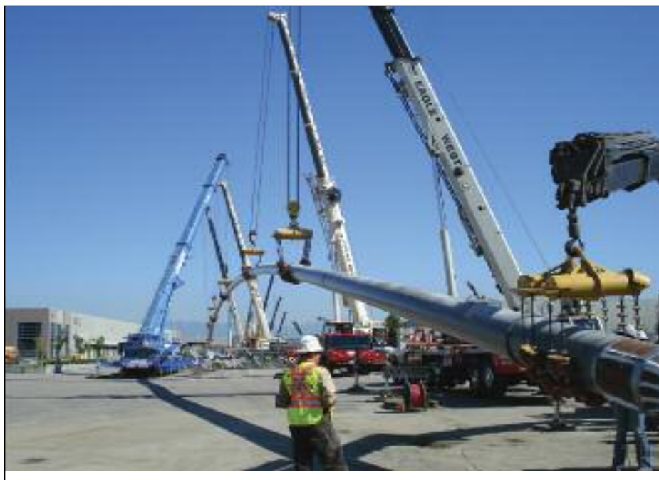
16 cranes were required to guide 1.4 kilometers of NPS 24 product line during installation.
