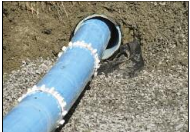
Fusible PVC offers the largest internal diameter of any sliplining material available today
