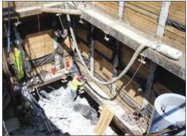
Entry shaft construction
