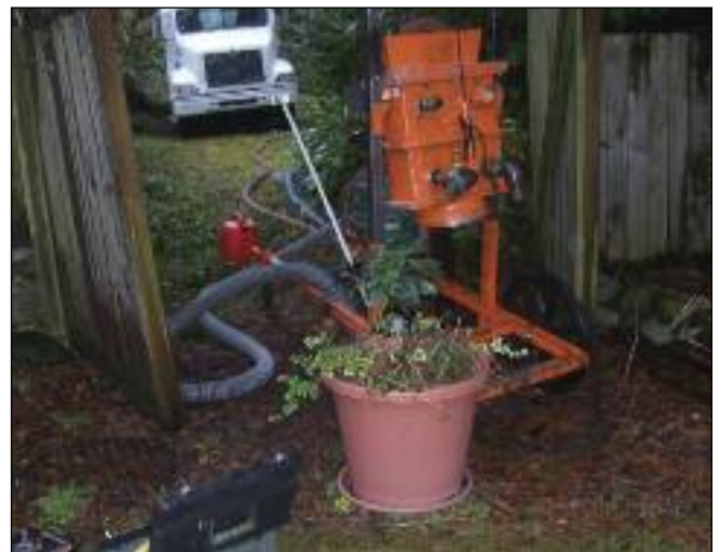
Mar-Tech's method of relining enables them to reline in more inconvenient areas
