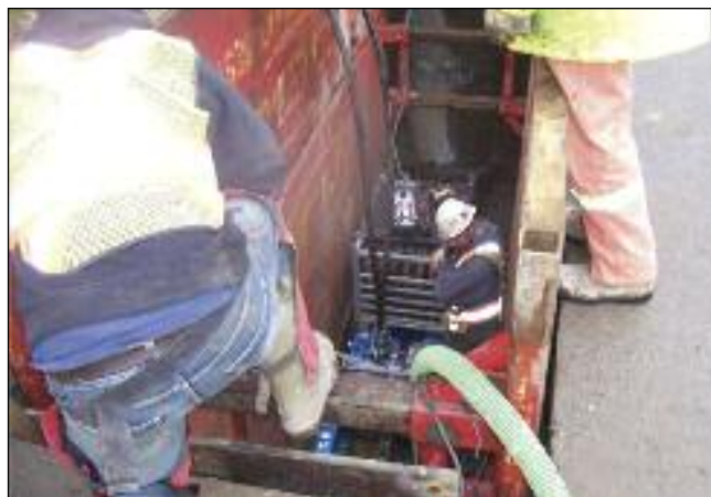
Tugging machine in trench with shoring cage
