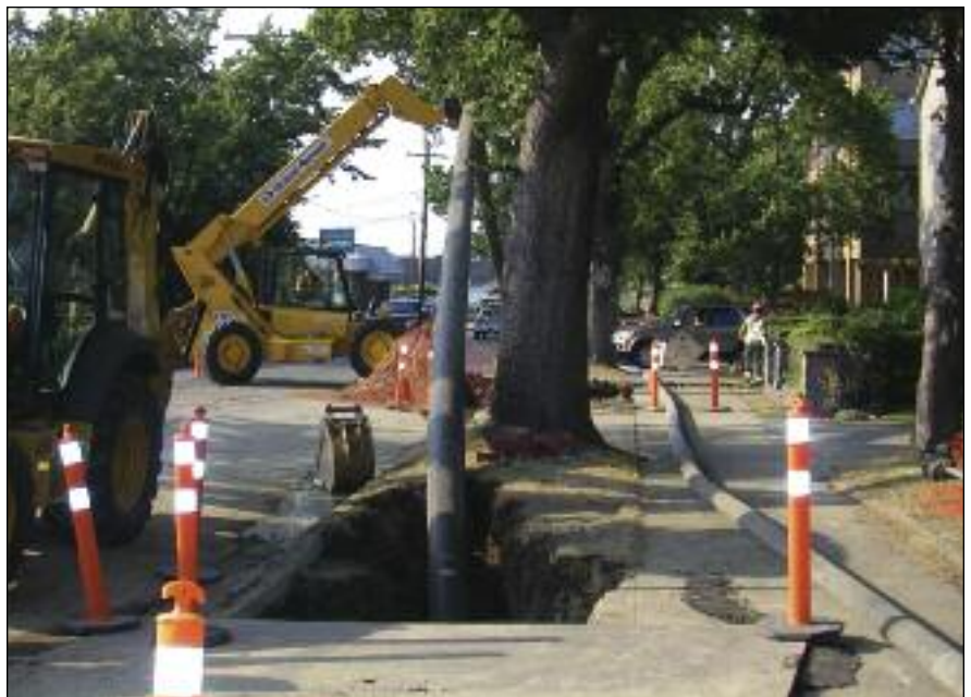
Figure 1 : Pipe Bursting Setup on Dallas Road for James Bay I&I Reduction Pilot Project
