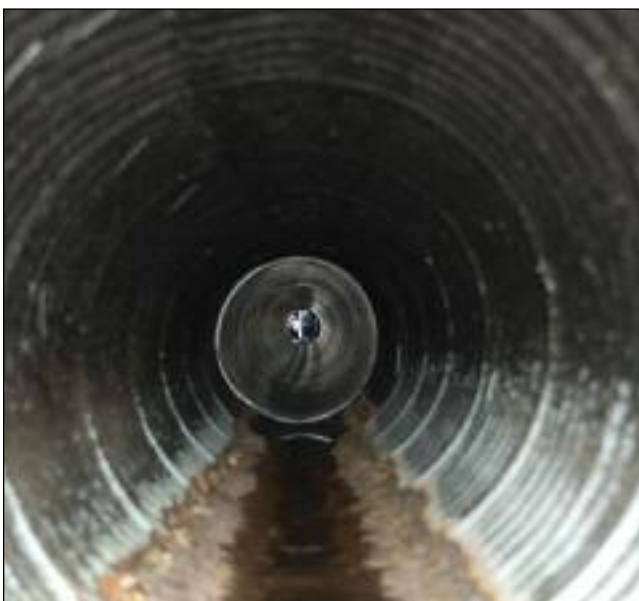
30" CMP before SPR™ rehabilitation
