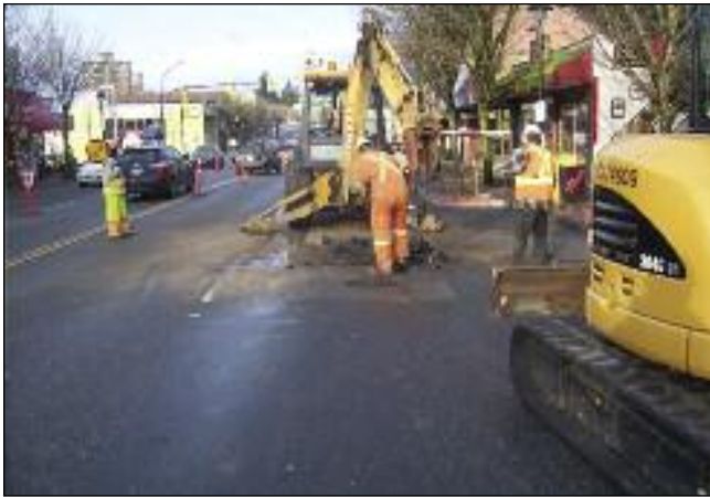
PW Trenchless replacing a manhole on Marine Drive.
