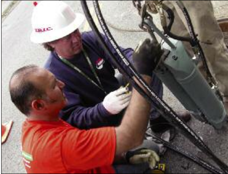
TRIC co-founder Ward Carter (hard hat) and client make adjustments to a 50-ton puller prototype
