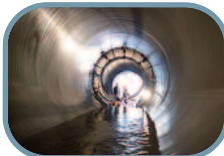
14' CMP Rehabilitation by SPR
