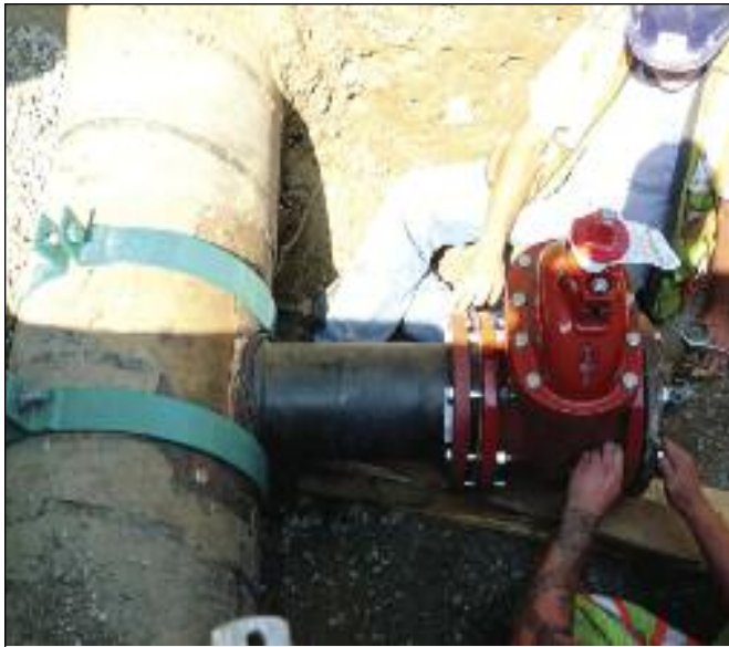
Branch watermain connection to the lined steel main
