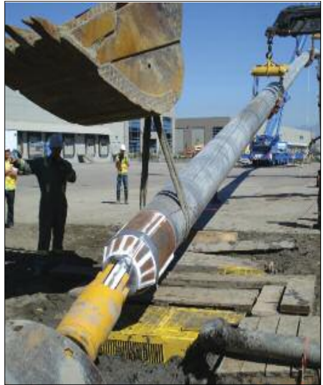
The NPS 24 product line is hoisted into position prior to product pull
