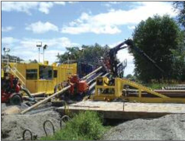
Rigging up Rig 4 in Richmond. More than 1.5 kilometers of inspected drill pipe sit ready for the pilot hole.
