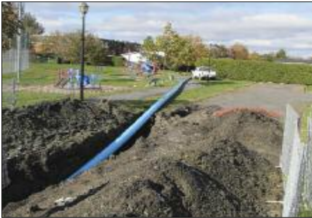
Use Fusible PVC in an HDD application for a more environmentally-friendly approach in areas like parks, lakes and rivers
