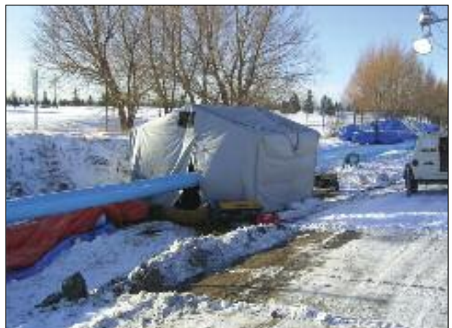
By using a weather shelter during the fusion process, Fusible PVC can be installed under any weather conditions
