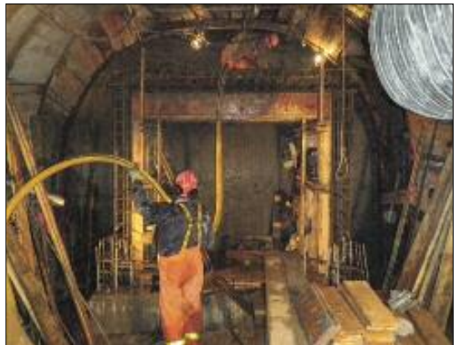
Construction of Tie-in Structure
