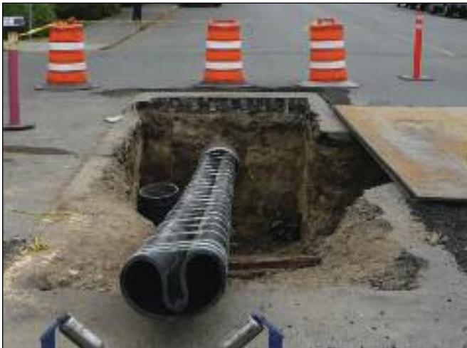
Typical pit size for liner insertion; remainder of the block untouched by construction activities
