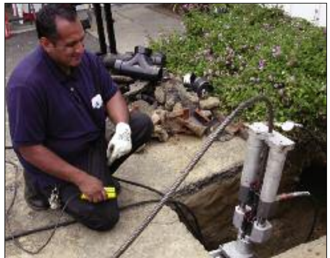
The original configuration of the TRIC lateral system is still widely in use today
