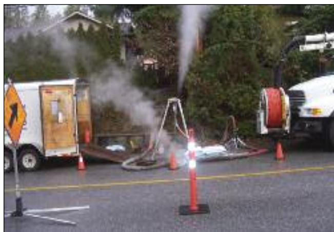
Steam curing of CIPP for shorter section of pipe in owner's backyard
