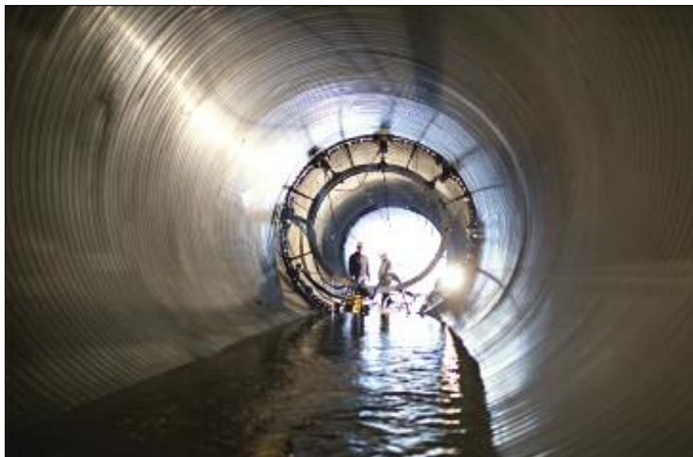
14' CMP rehabilitation by SPR™
