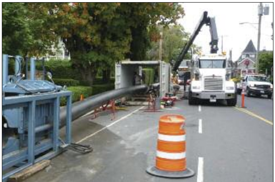
Pipe fusion and folding site on the roadside
