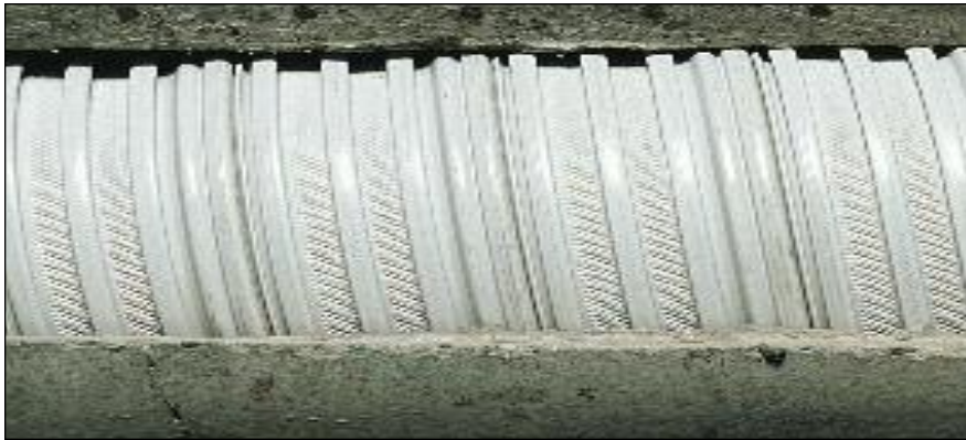
SPR EX™ (expanded against host pipe)
