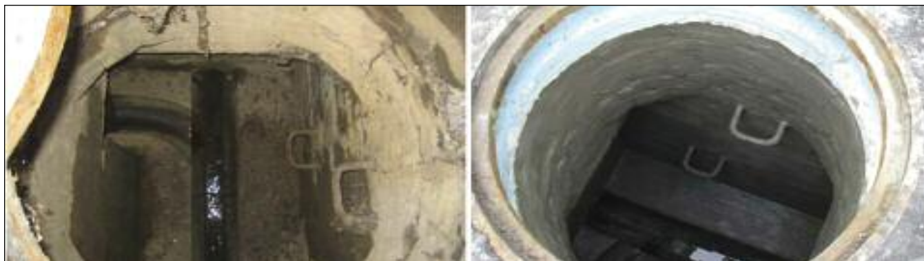
Figure 6: Before and after manhole coating and lining
