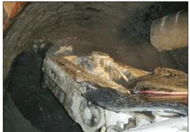
Tunnel face – roadheader in action
