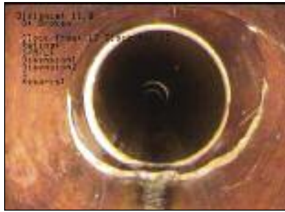
Figure 4: Even though the pipe is broken, it can be lined as the shape is still circular
