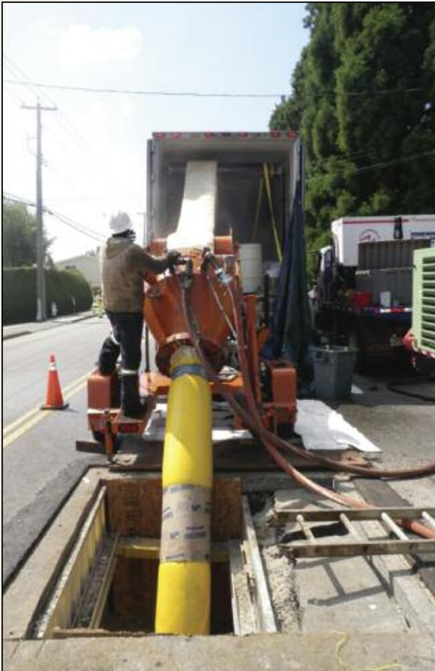
Inverting the liner
