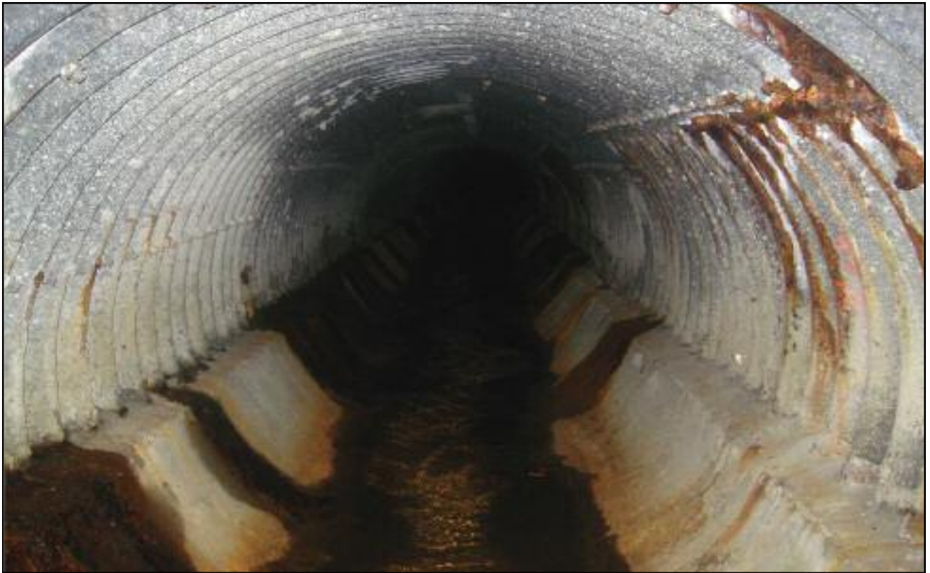
Deteriorated 1,800 mm CSP culvert selected for slip lining with HDPE
