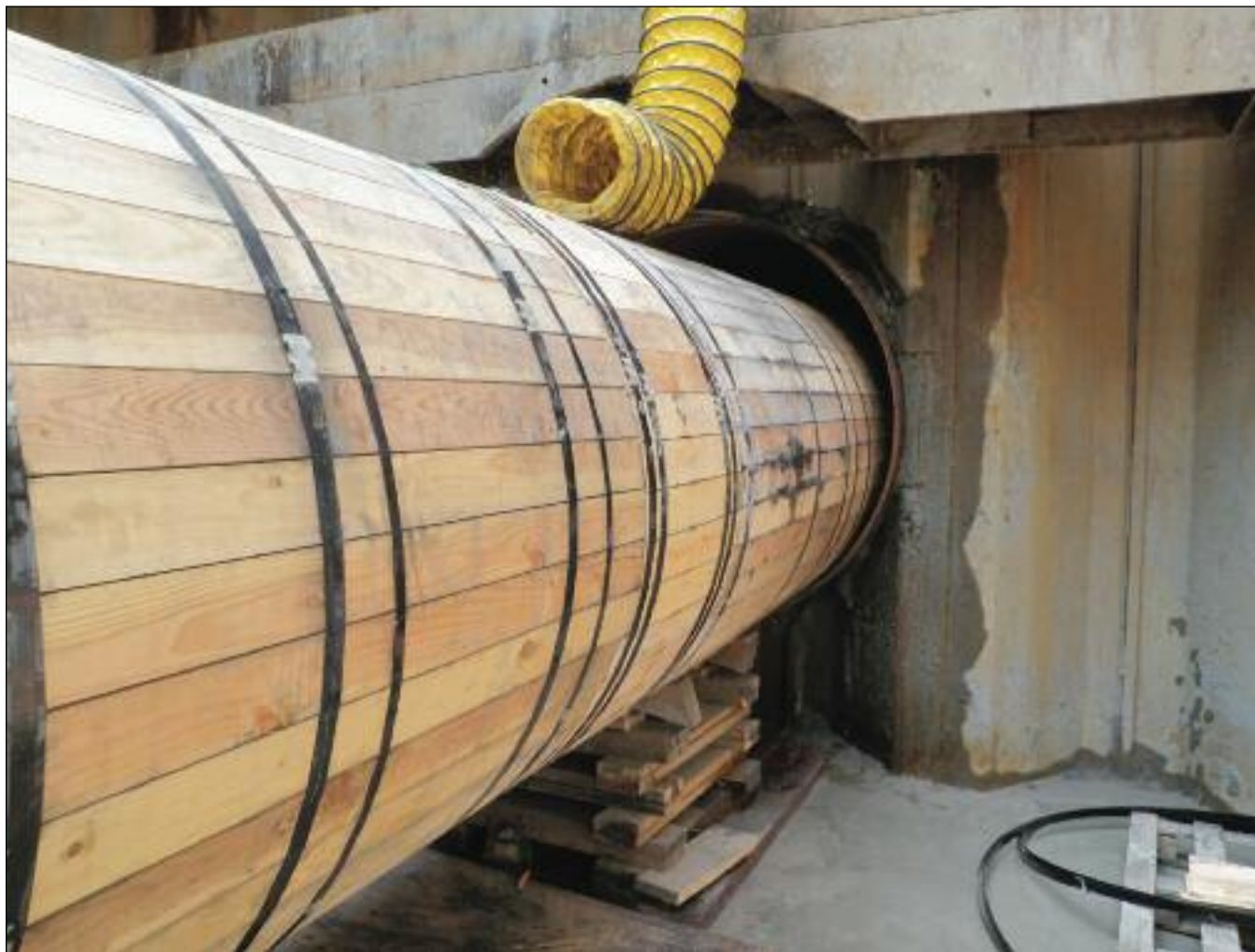
Installation of wood-lagged carrier pipes
