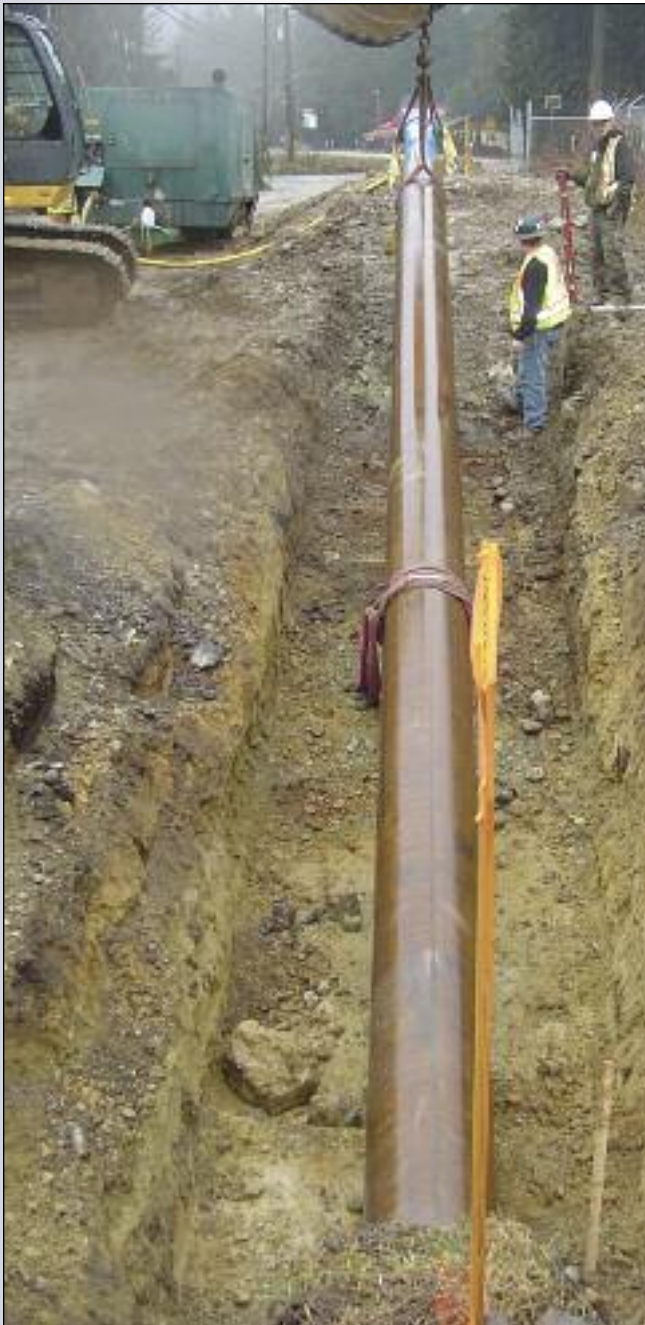
First section of casing in Harrison River crossing project
