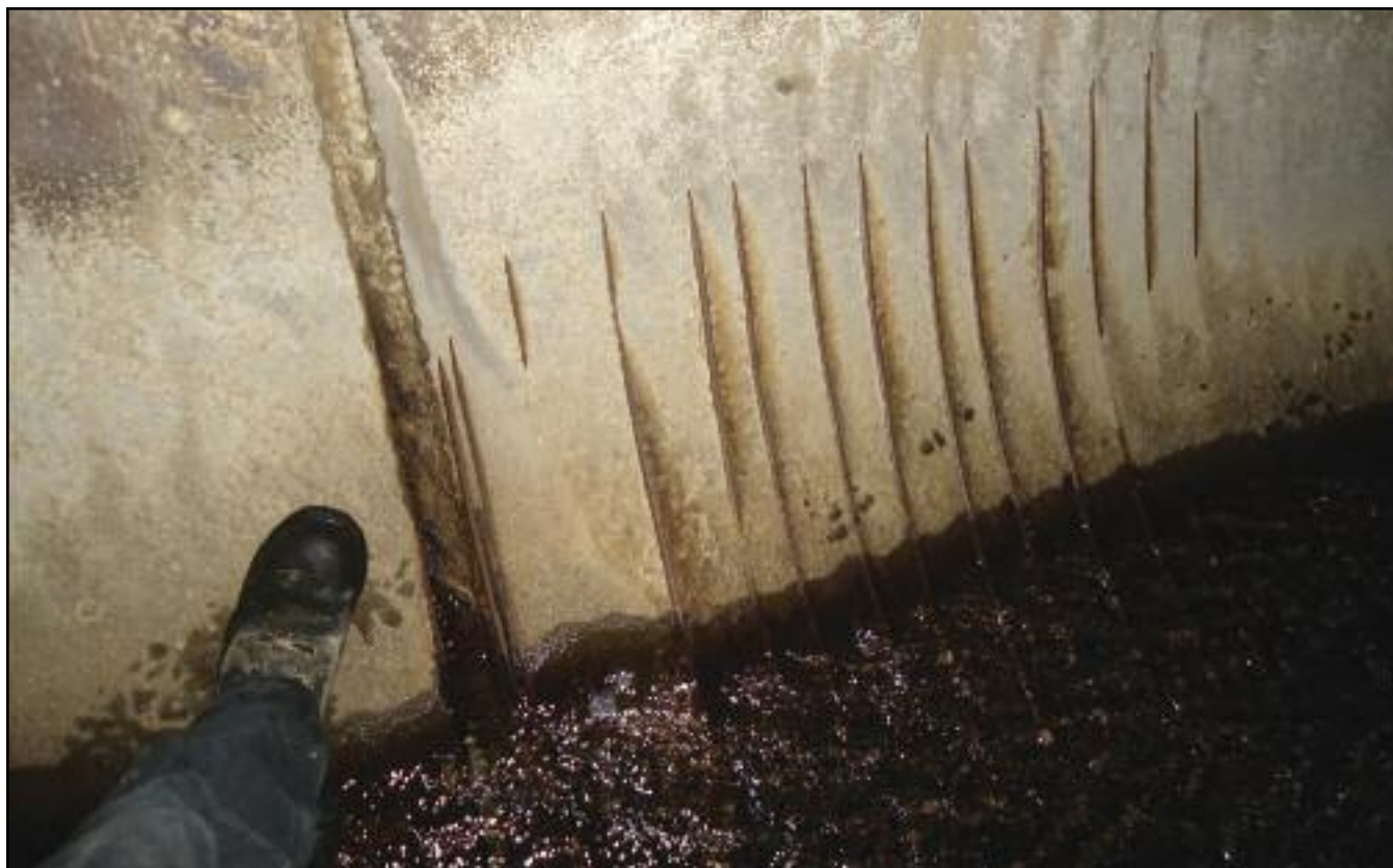
1,800-mm circular concrete culvert with loss of concrete cover over steel reinforcement
