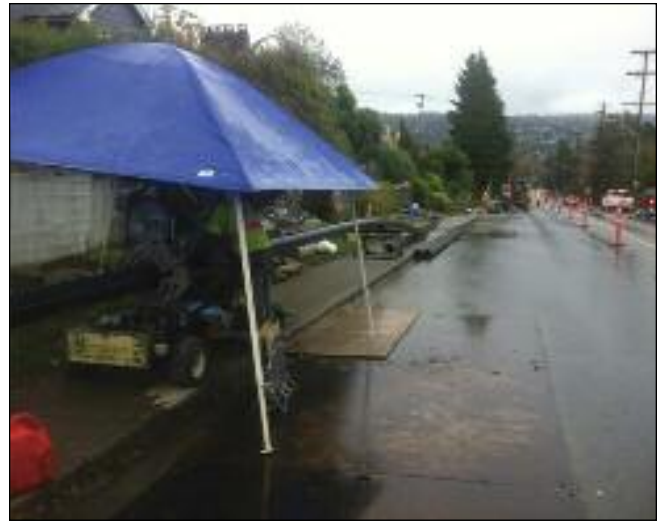
Fusing HDPE pipe
