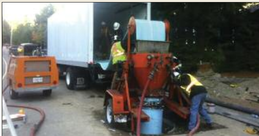
Liner installation in the Whistler Alta Vista project
