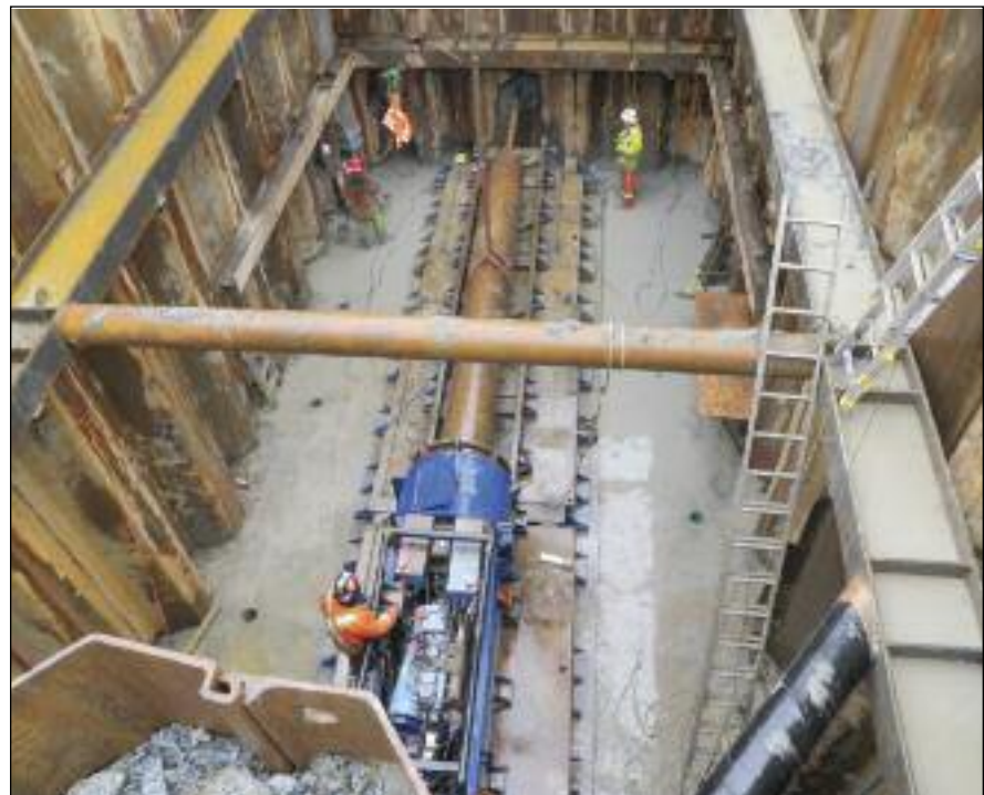
Installation of 600-mm casings following 100-mm pilot tube
