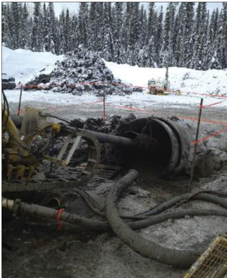
Installation of casing started in December 2012
