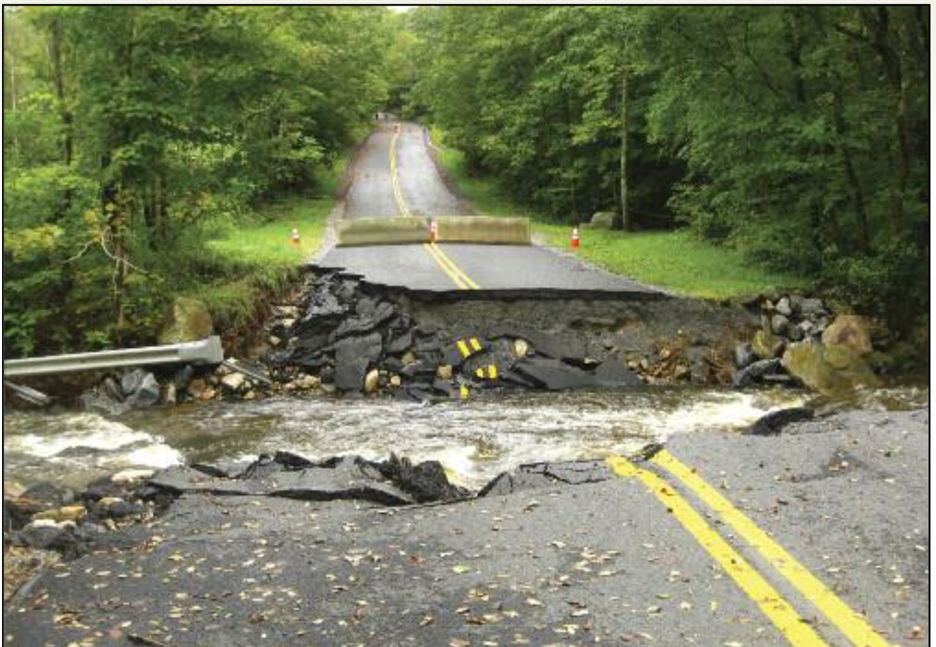
Road closure caused by culvert failure in Massachusetts [Photo by Massachusetts River Alliance]
