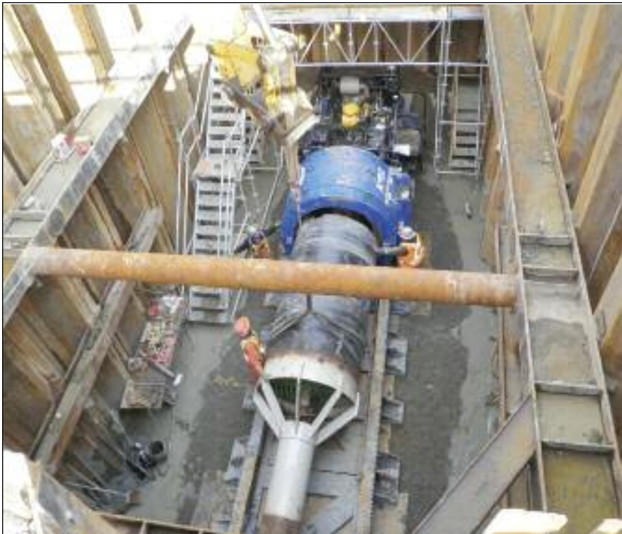
Installation of 600 mm to 1700 mm expander
