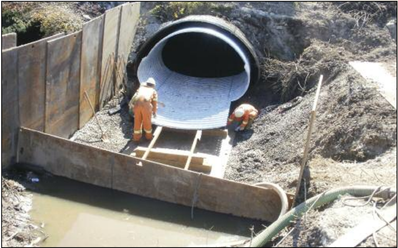
A Bolt-A-Plate structure system was used to slipline a culvert under a BC Rail track.
