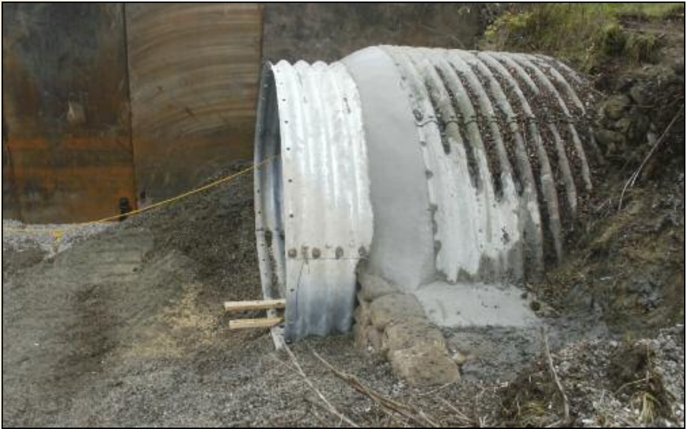
A dry working environment was required for the culvert rehabilitation project.
