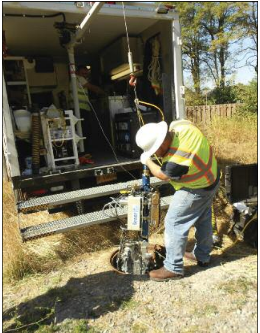
The SewerVUE Surveyor robot is deployed at St. Johns manhole 28-377.
