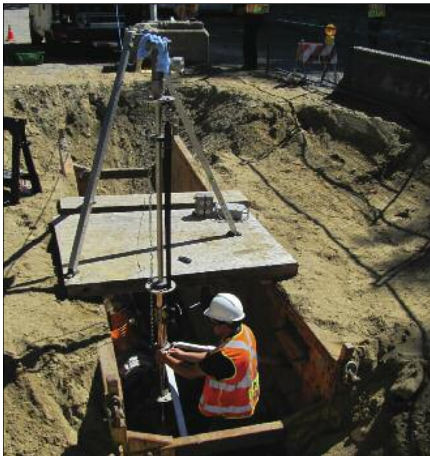
Water service continued as inspection of the main was conducted.
