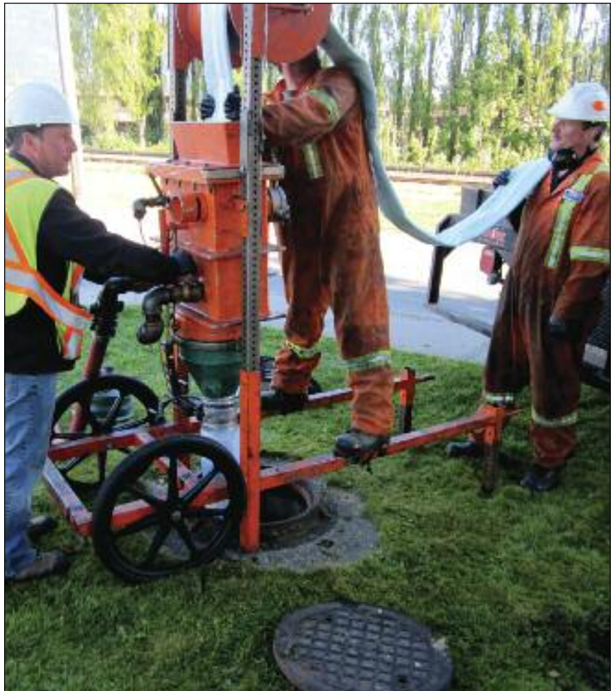
Mar-Tech installs liner before curing.
