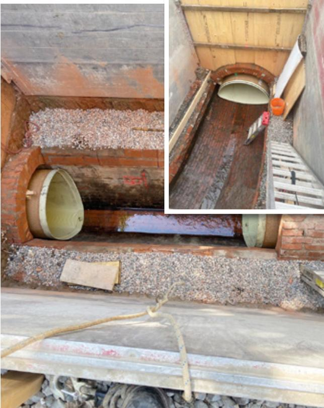
*Each 2.4m segment of GRP was carefully pushed together for a watertight joint*
