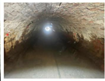
*Condition of the crown put this section high on the City's rehab priority list*
