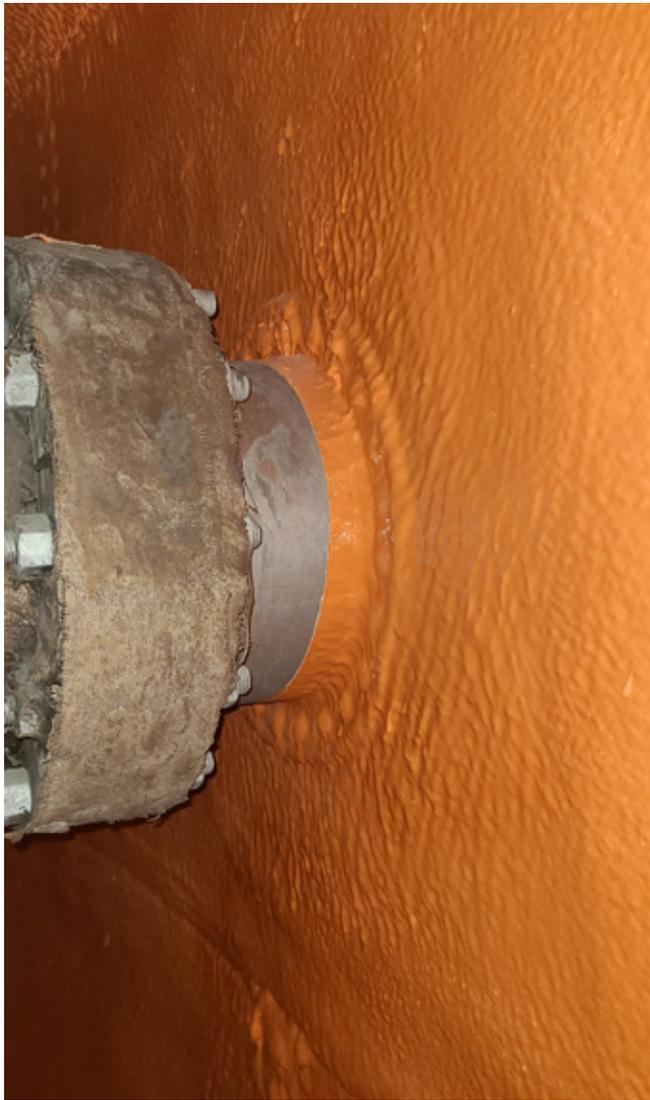
*Detail of coating termination against the uncoated utilities*
