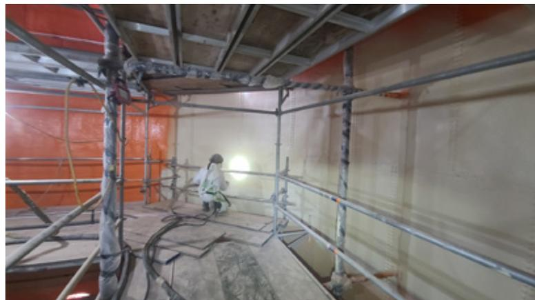
*The OBIC system utilizes a structural version of spray foam insulation as a middle layer*
