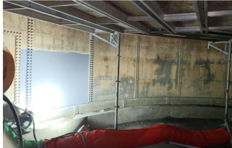
Tanks walls were corroded with serious pitting
