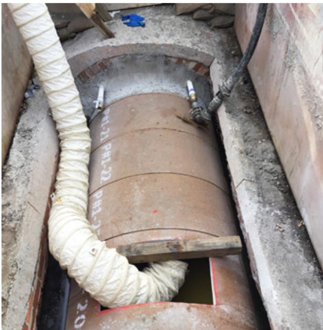
Annular grouting completed the construction process
