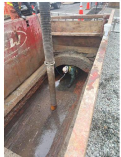
*Brick pipes cleaned out using high pressure water, and debris removed by hydrovac*
