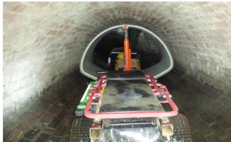
*Each GRP segment was maneuvered into place using an electronic motorized cart*
