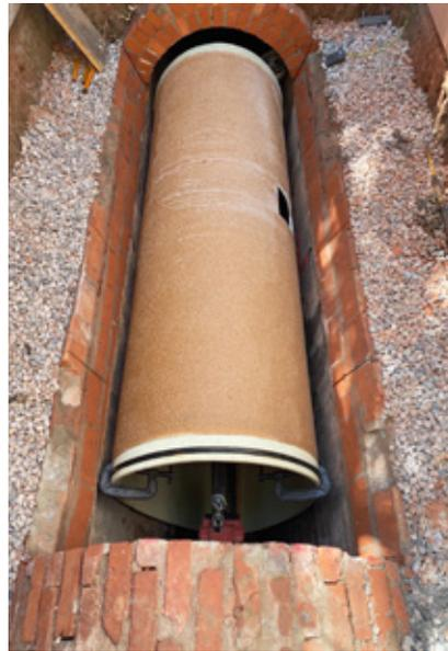
GRP segments are treated with bonded graded aggregate material to enhance adhesion to the annular grout
