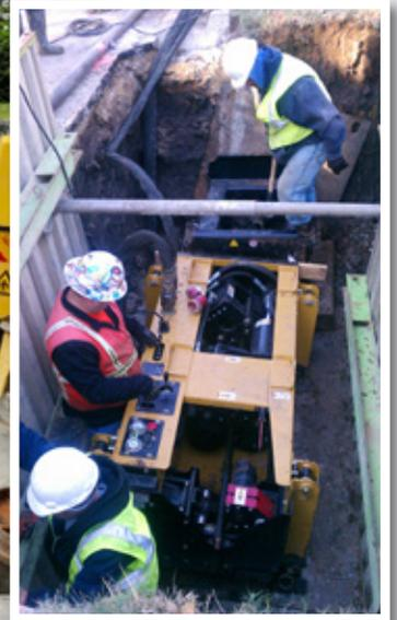
*Typical pipe bursting setup*
