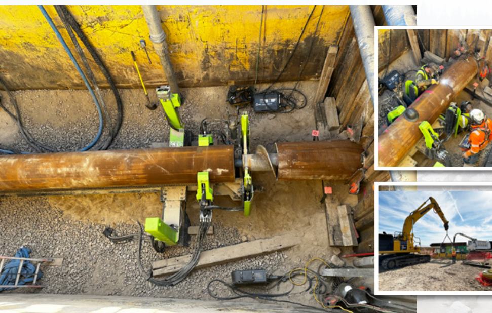
Boise ID project installed 300 feet of 24-inch casing for electrical conductors under parallel road and railway
