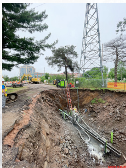
EBI Drilling utilizes their HZR220 to install 100 feet of 6-inch steel casing below railroad tracks in less than 8 hours. Before an additional 160 feet the next day
