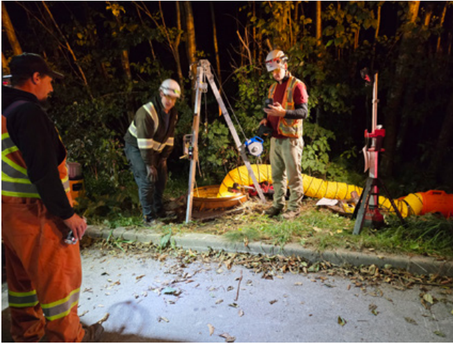
Manhole rehab work was performed with quick and mobile short-duration site setups
