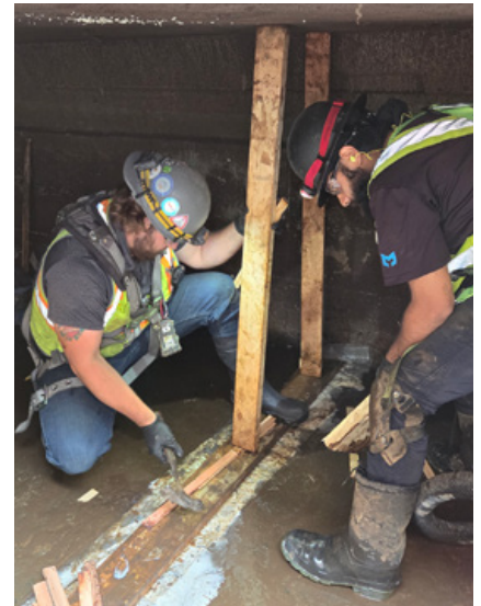
Strutting placed on floor joint after application of resin and oakum
