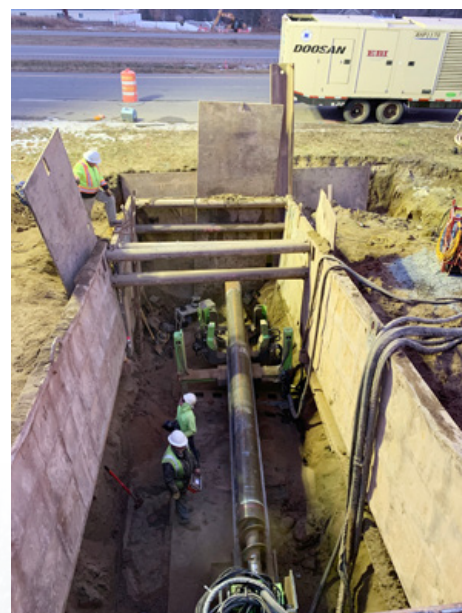
From the Launch Pit: EBI's operator uses the GEONEX wireless remote control to operate their HZR610 Drill machine for a 320-foot installation below the highway
