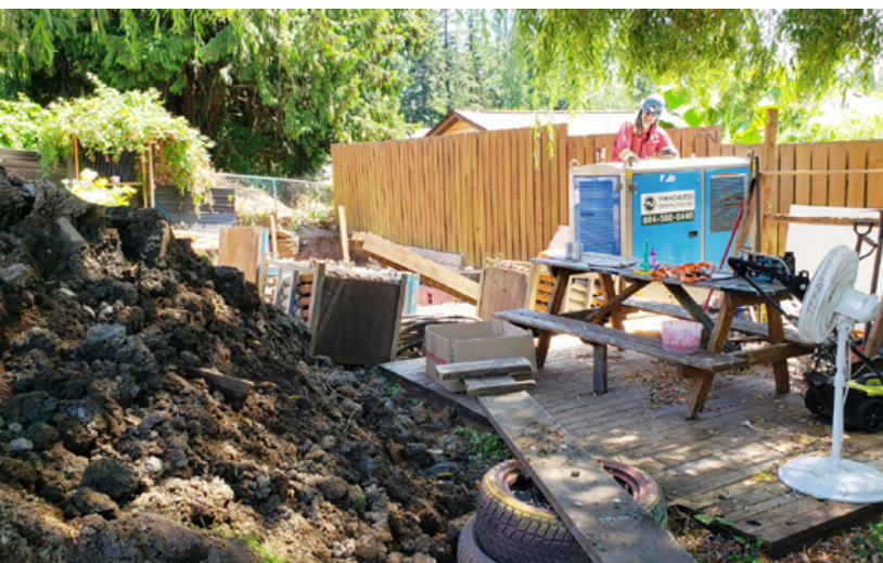
Small footprint of pipe bursting rigs helped navigate around the backyard clutter
