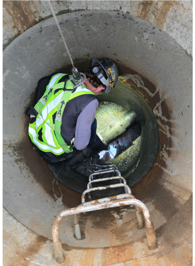
Full condition assessment and mapping of the wastewater system prior to installation
