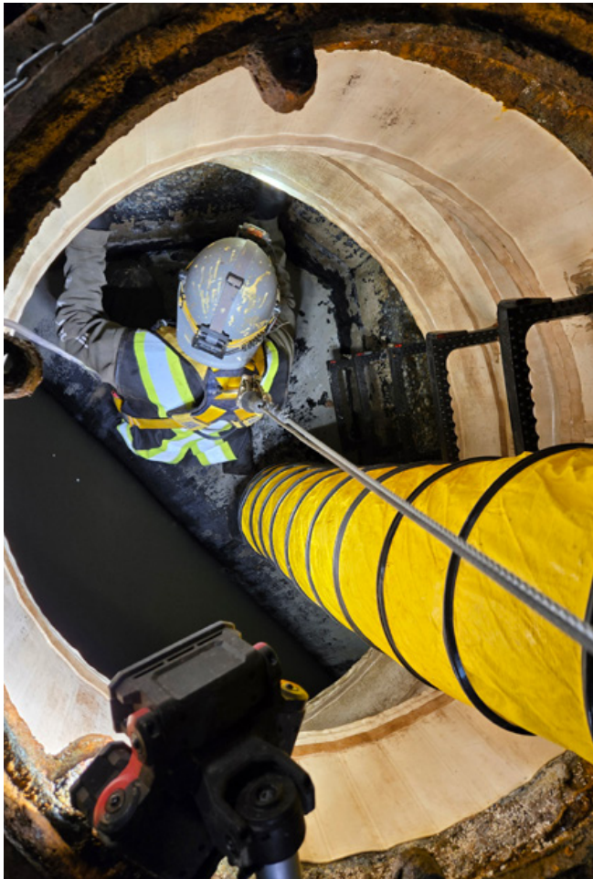
Factory-certified crews sealed active leaks, rebuilt compromised structures, and optimized benching
