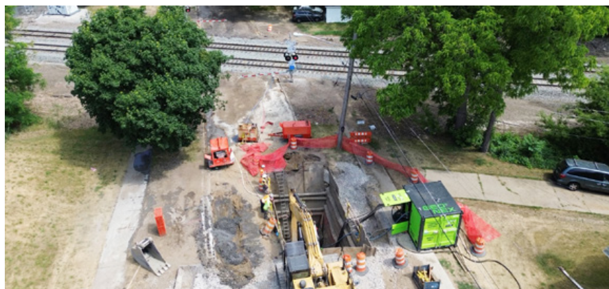
Aerial view of equipment set up to bore under the high speed Amtrak railway
