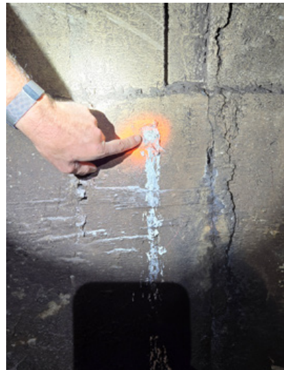
Close up of grout return
