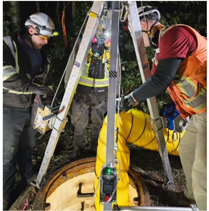
A targeted rehabilitation program using polyurethane injection and cementitious restoration was implemented
