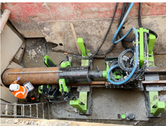
Technician uses the remote control to operate the GEONEX HZR610 drill machine set up for 10-foot casing lengths
