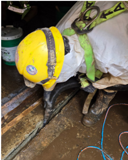
Floor joint cleaned out then stuffed with oakum
